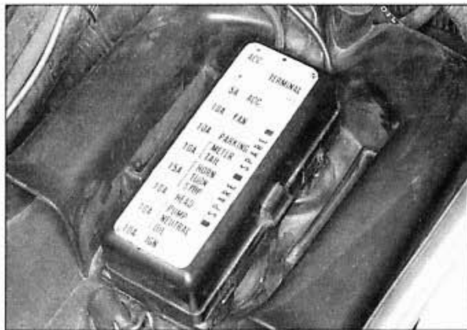
5.1a The accessory fuses are beneath a cover inside the top compartment . . .
